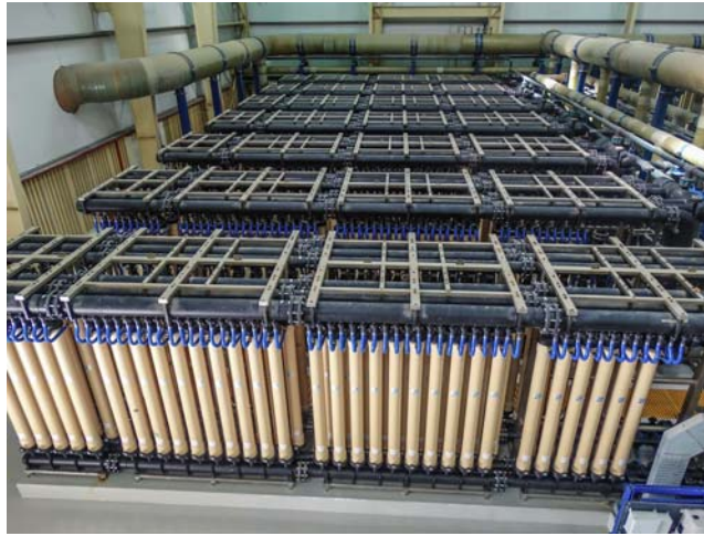
FIGURE 9.3 Pressurized membrane filtration system with vertical membrane elements.
