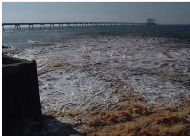
FIGURE 10.1 Discharge of untreated backwash water from granular media filters.
