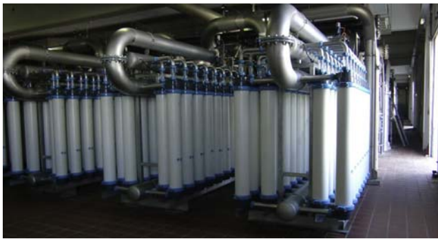
FIGURE 9.8 Pentair X-Flow Seaflex ultrafiltration pretreatment system.
