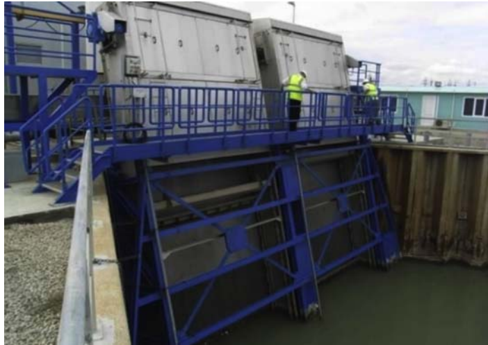
FIGURE 5.2 Coarse screens of onshore intake.
