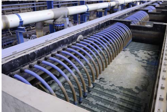
FIGURE 9.2 Ultrafiltration (UF) pretreatment system of the Adelaide desalination plant, Australia.
