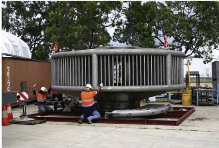
FIGURE 4.10 Steel offshore intake tower.
