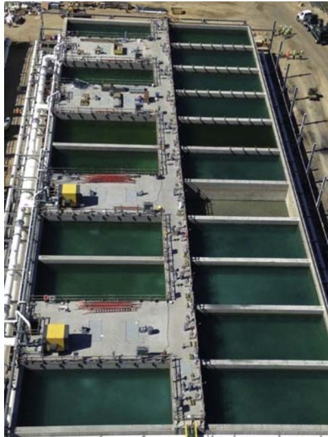
FIGURE 8.3 Single-stage gravity filters of the Carlsbad desalination plant, California.
