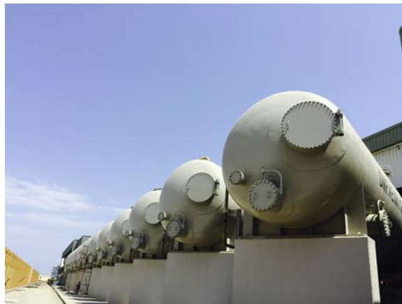
FIGURE 8.5 Horizontal pressure filters—Al-Ghubrah desalination plant, Oman.
