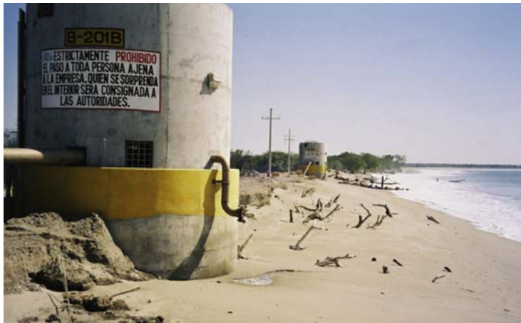
FIGURE 4.3 Two Ranney wells for Salina Cruz SWRO plant, Mexico.
