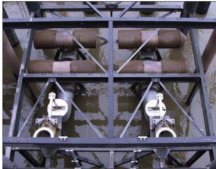
FIGURE 5.6 Wedge-wire screens of Beckton desalination plant, London, UK.
