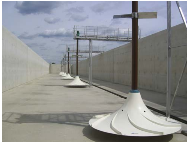
FIGURE 6.2 Flash mixers in coagulation tank.
