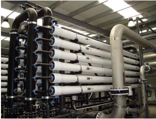
FIGURE 9.7 Pentair X-flow Seaguard ultrafiltration pretreatment system.
