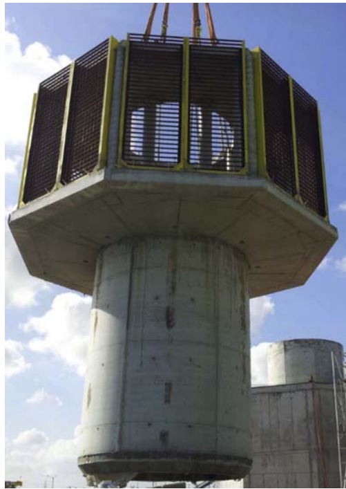
FIGURE 5.1 Vertical intake tower with coarse screen.
