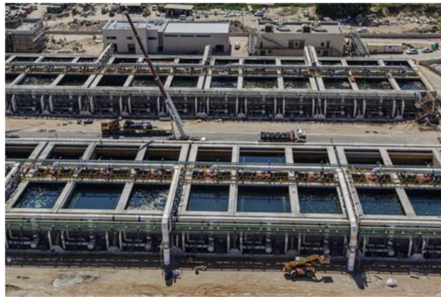
FIGURE 8.4 Single-stage gravity filters of the Sorek desalination plant, Israel.
