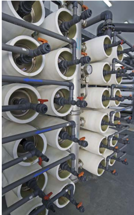
FIGURE 3.6 Membrane pressure vessel sampling ports.
