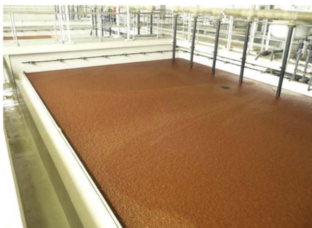
FIGURE 7.5 Sludge layer on the surface of DAF clarifier.
